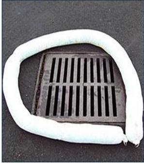
Place 8 ft. absorbent sock around basin to prevent spilled fuel from entering
