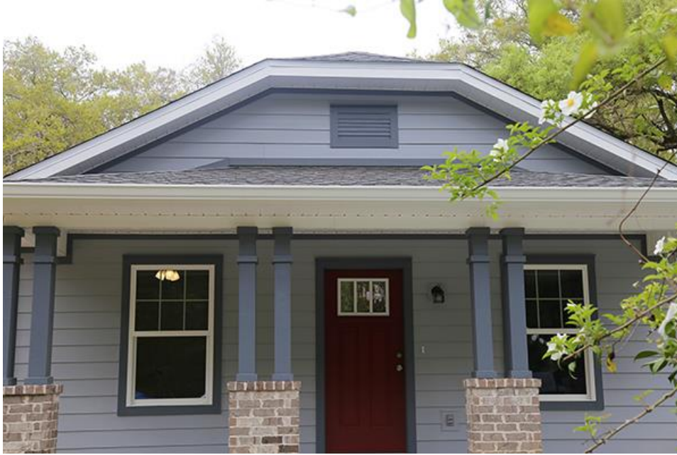
Escambia County resident Estella Marshall's new home, which was constructed through the county's Housing Demo and Replacement Programs.
