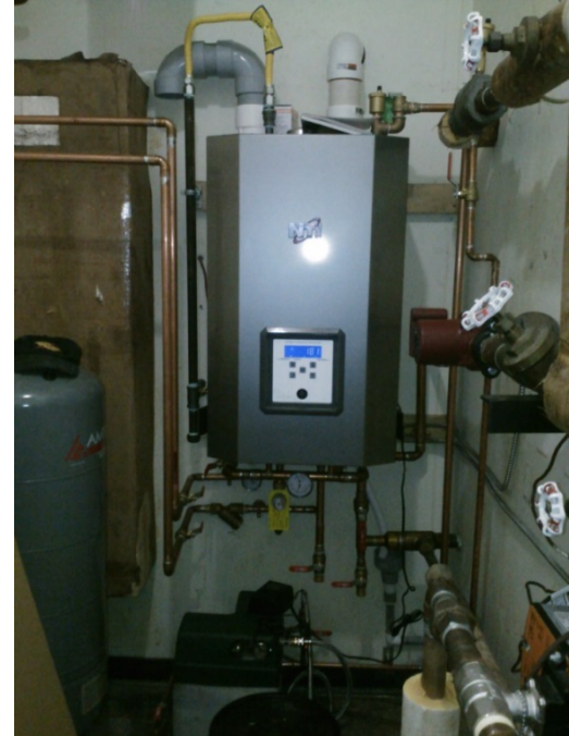
New, wall mounted, high efficiency propane boiler
