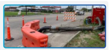
The lane closure on Loop 197 at 19th St. is due to the on-going rehabilitation of the adjacent sanitary sewer lift station. The lift station had to be bypassed in order to maintain sewer service to the area while performing the work. Therefore, temporary sewer piping had to be installed in the manhole located in the closed lane. Unfortunately this project is not scheduled for completion until the end of May at the earliest.
