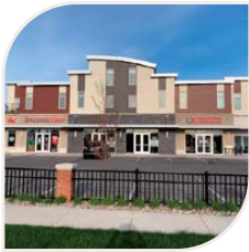
CAMPUS COMMONS 16,000 square foot mixed use retail & residential
