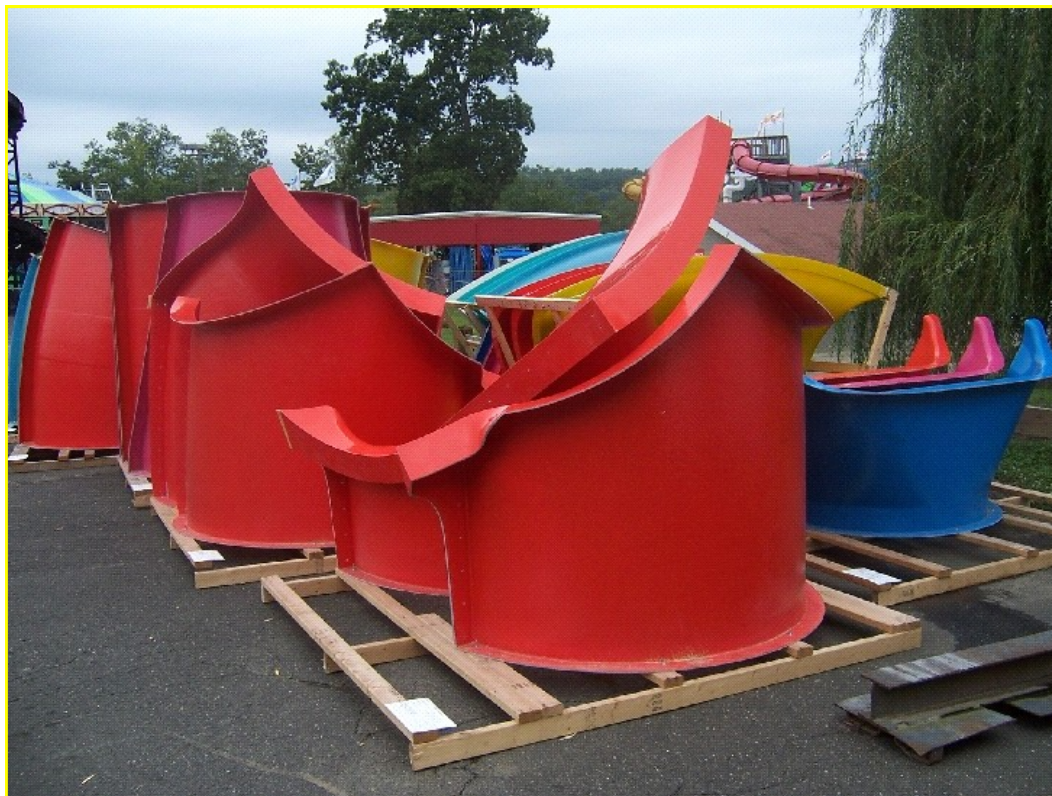
Fiberglass sections of the new waterslides being installed at Quassy Amusement & Waterpark wait to be assembled. (Quassy photo)
