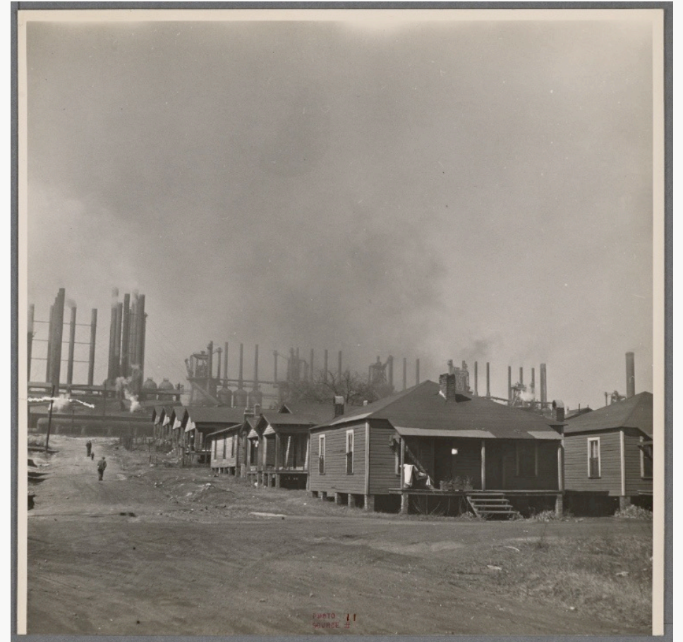
Steel mill and workers' houses near Birmingham, Alabama- 1937 ( https://digitalcollections.nypl.org/items/ba309cea-955e-4288-e040-e00a18066c61 )
