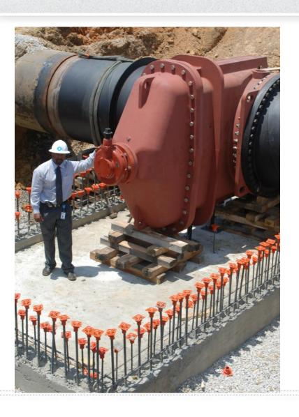
60-inch diameter **American Flow Control resilient** seated gate valve. **Installed** horizontally because it's more than 13 feet tall vertically. Weight is 29,854 pounds; 984 turns to open or close.
