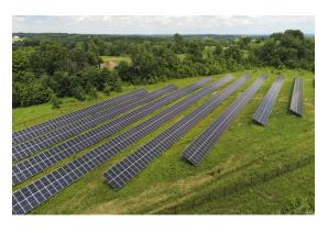
Fixed tilt ground mounts are typically angled at 25 degrees. With no moving parts, they are usually the most cost effective under 2 MW and easy to maintain.
