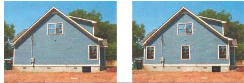
The image on the left shows a side elevation with a large expanse of wall without windows or other details. The image on the right shows the same elevation if several additional windows were added.
