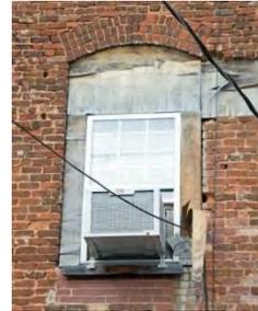
**Example of window AC unit inappropriately installed on front façade resulting in replacement and alteration of original window framing.**
