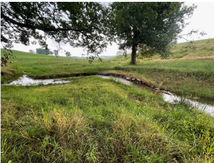
Figure 3. Wet-weather seep before being armored with rocks resembling riprap along Ruby Run's streambank in Preston County, West Virginia, USA.
