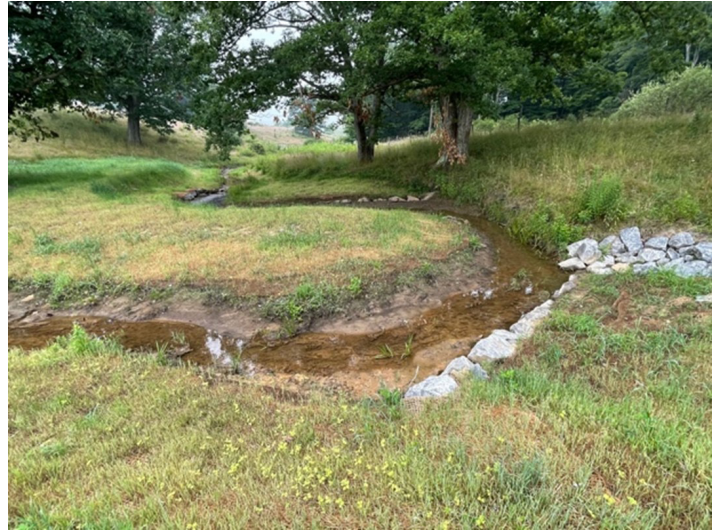
Figure 4. Log vanes, rocks vanes, point bar, and rocks resembling riprap along Ruby Run's streambank, Preston County, West Virginia, USA.
