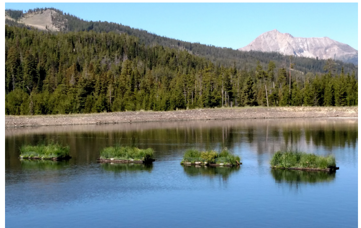
FIGURE 4. BioHavens located in a high-elevation wastewater pond near Big Sky, MT, one year after installation.
