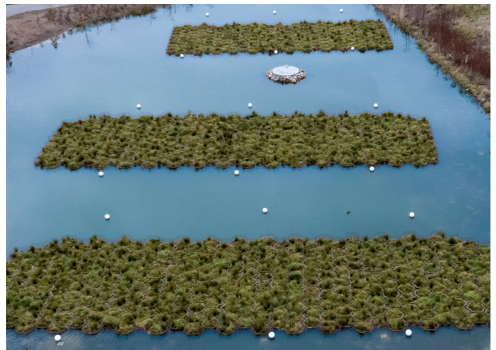
FIGURE 14. PhytoLinks FTW installation Brampton, Ontario Canada (2017) showing 6 anchor lines (white buoys) per grouping of modules.
