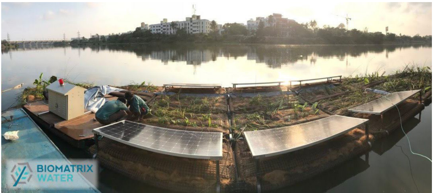
FIGURE 9. Floating island with solar power to drive aeration through submersible Venturi aerators all managed and powered completely onboard the island with GSM remote controls and monitoring.
