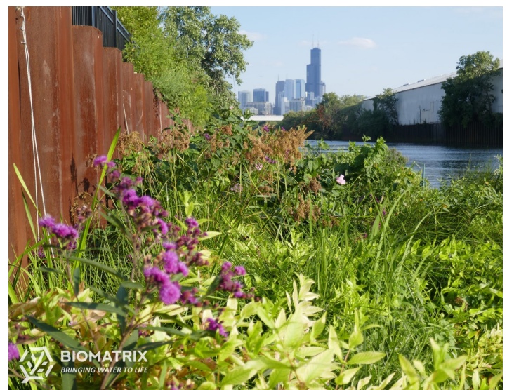
FIGURE 7. Floating riverbank – part of “Wild Mile Chicago” in the United States. (See https://www.wildmilechicago.org/about-us for additional information.)
