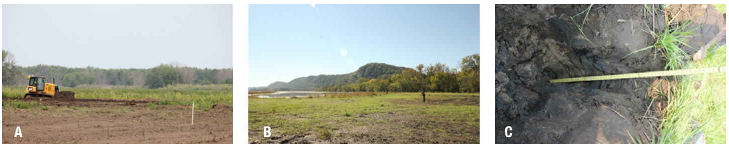
Figure 6: Post construction conditions (a,b) at the Conway Lake HREP, where fine grained soils (c) were incorporated into the wetland project design. (Source: USACE St. Paul District.)
