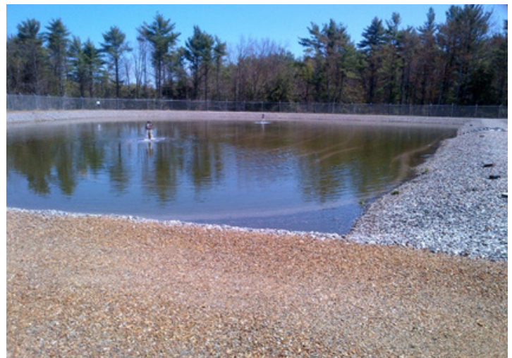
Figure 3. Franklin Pierce University Rapid Infiltration Bed, south basin.
