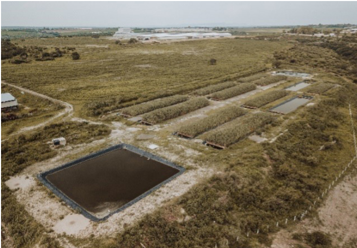
Figure 3. Examples of horizontal subsurface flow wetlands (HSSFW) for water treatment. On left, a 7,500 m 2 full-scale HSSFW located in Jalisco, Mexico, planted with Reed ( Phragmites australis ), designed for treating up to 900 m 3 of industrial wastewater, constructed by Soluciones Ecológicas del Desierto S.A. de C.V. (Photo reproduced with permission of Soluciones Ecológicas del Desierto S.A. de C.V.) To the right, a full-scale HSSFW installed in Ponte de Lima, Portugal, and planted with Canna flaccida , Canna indica , Zantedeschia aethiopica , Agapanthus africanus , and Watsonia borbonica . (Photo by Cristina Calheiros)
