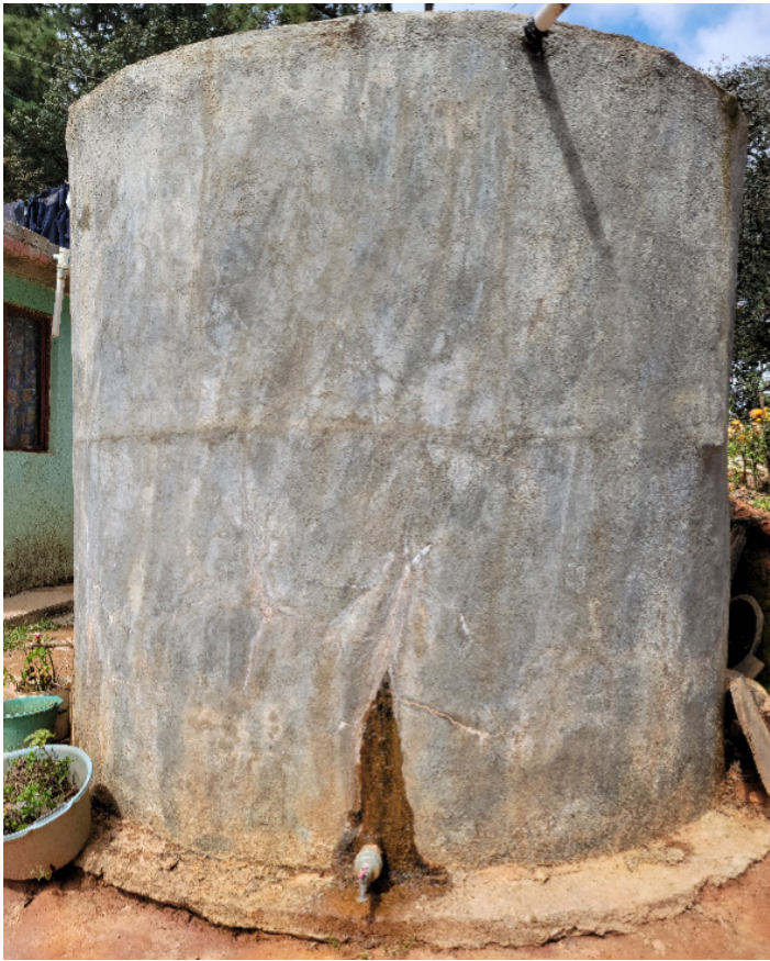
Figure 2. A concrete cistern, use for rainwater harvesting from the roofs of homes in El Éden, Sierra Gorda Biosphere Reserve, Mexico. This one was leaking a bit around the faucet, but the owners did not want to repair it yet, because the wasps living by their home used that spot for drinking. (Photo by Marinus Otte)
