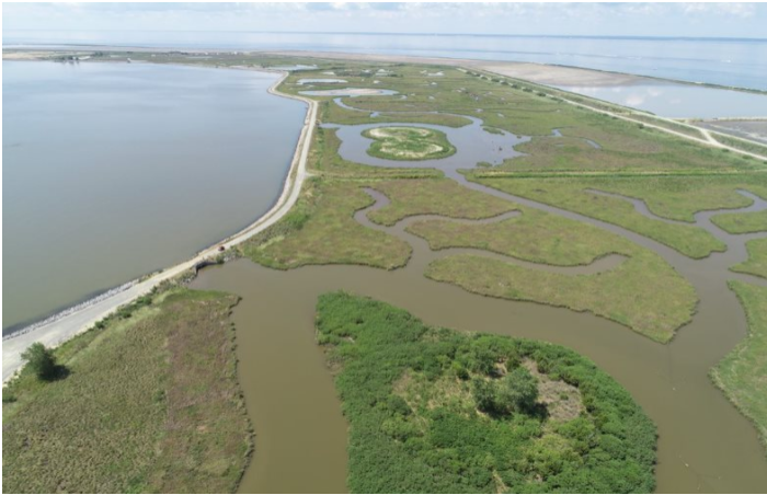
FIGURE 3. Aerial view of Cell 2 (MDOT MPA).
