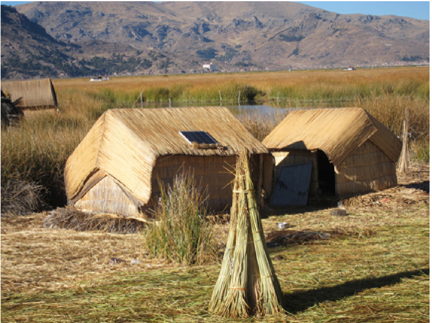
Figure 5. House built of totora reeds. (Photo: tillthemoneyrunsout.com)
