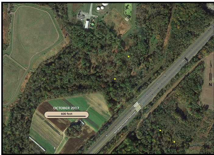
FIGURE 20. The wetlands constructed in the Assiscunk riparian corridor do not have complex or complicated water control structures and fit well into the surrounding landscape. Having been in place for nearly 30 years and now supporting a predominance of native species common in the riparian corridor, the constructed wetlands are nearly impossible to distinguish from other “natural” wetland depressions found within and along the stream corridor floodplain. Yellow dots pin-point four areas of constructed wetlands built between 1988 and 1993; the two upper ones are the subject of this article.
