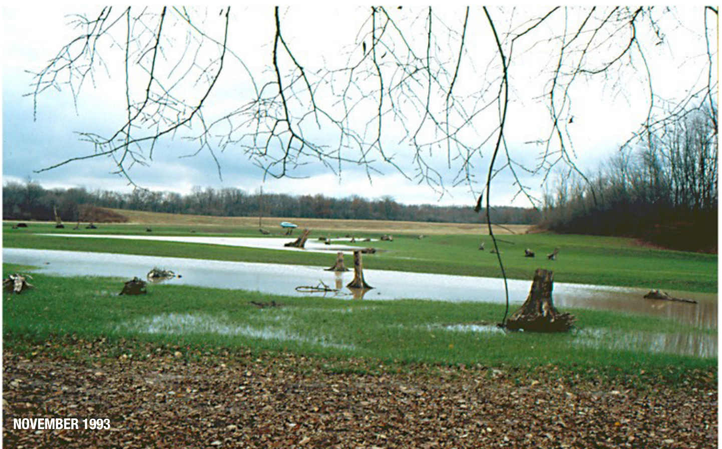
FIGURE 6. Following finish grading, stumps and other woody debris were placed to create escape cover for amphibians and singing/sentry platforms for various birds. The final task prior to onset of winter conditions was to protect the wetland from erosion. A combination of oats and annual ryegrass was seeded to provide rapid cover of the site. Effective as protective cover, these grasses did not compete with colonizing hydrophytes and soon succumbed to inundation. Yet, remnant stems and leaves acted to catch and hold “seed rain” from spring flooding in 1994 and to add detrital organic matter and nutrients to the soil substrate.
