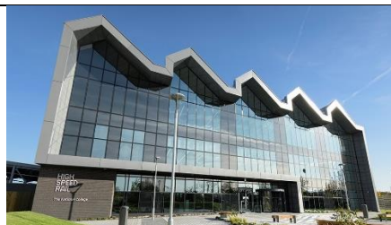
Advanced Transport and Infrastructure National College
