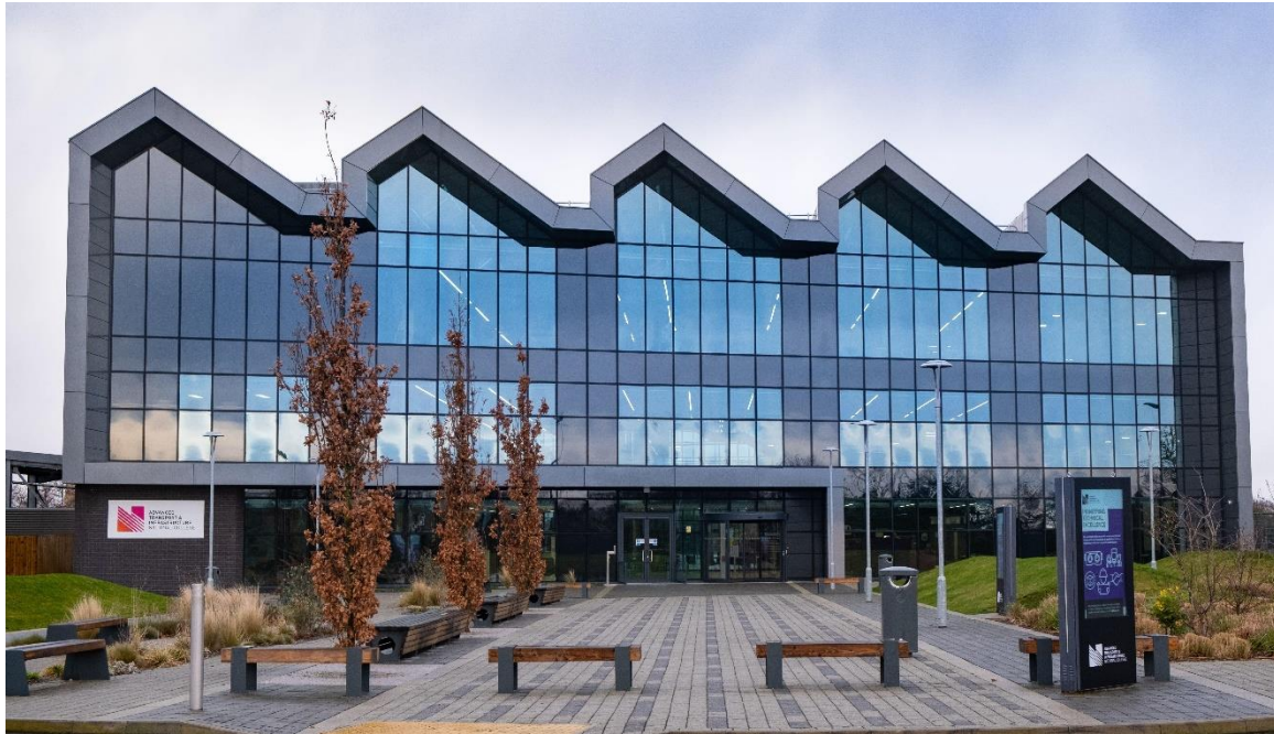
41) The National College for Advanced Transport & Infrastructure: A purpose-built facility to train the next generation of high-speed railway practitioners. Facilities include a full-size high-speed engine and track section to learn first-hand skills.
