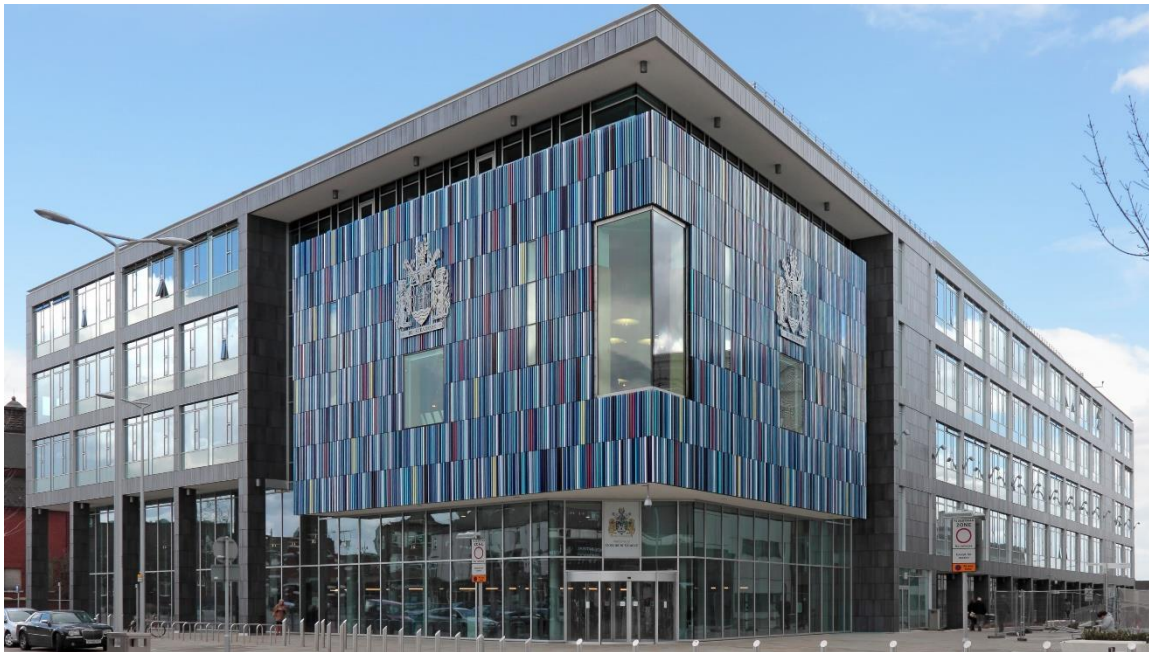
1) Doncaster Council Office, Civic & Cultural Quarter: The modern and distinctively designed five-story office complex, opened in 2013, houses most of the Council's services on one central site and includes a purpose-built customer service centre.
