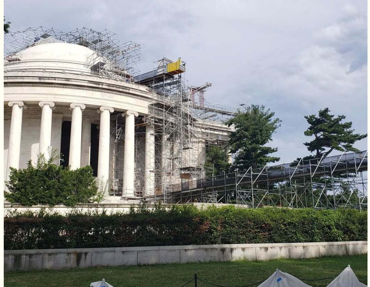
Roof replacement at the Thomas Jefferson Memorial
