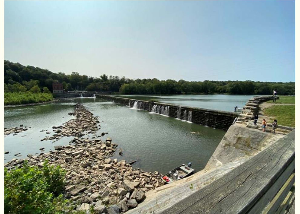
Dam repair at the C&O Canal National Historical Park
