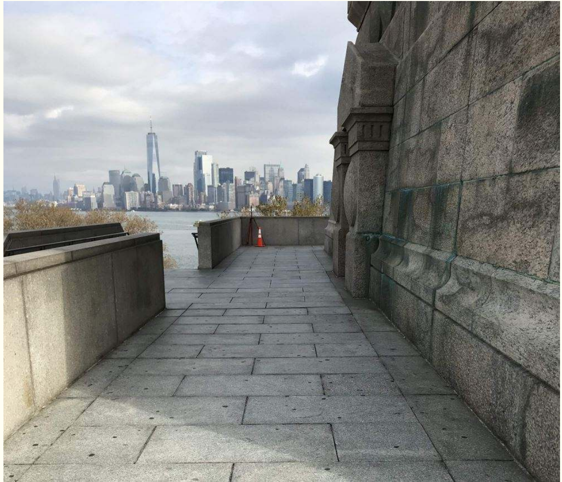
Rehabilitation of the Terreplein Plaza, Statue of Liberty National Monument
