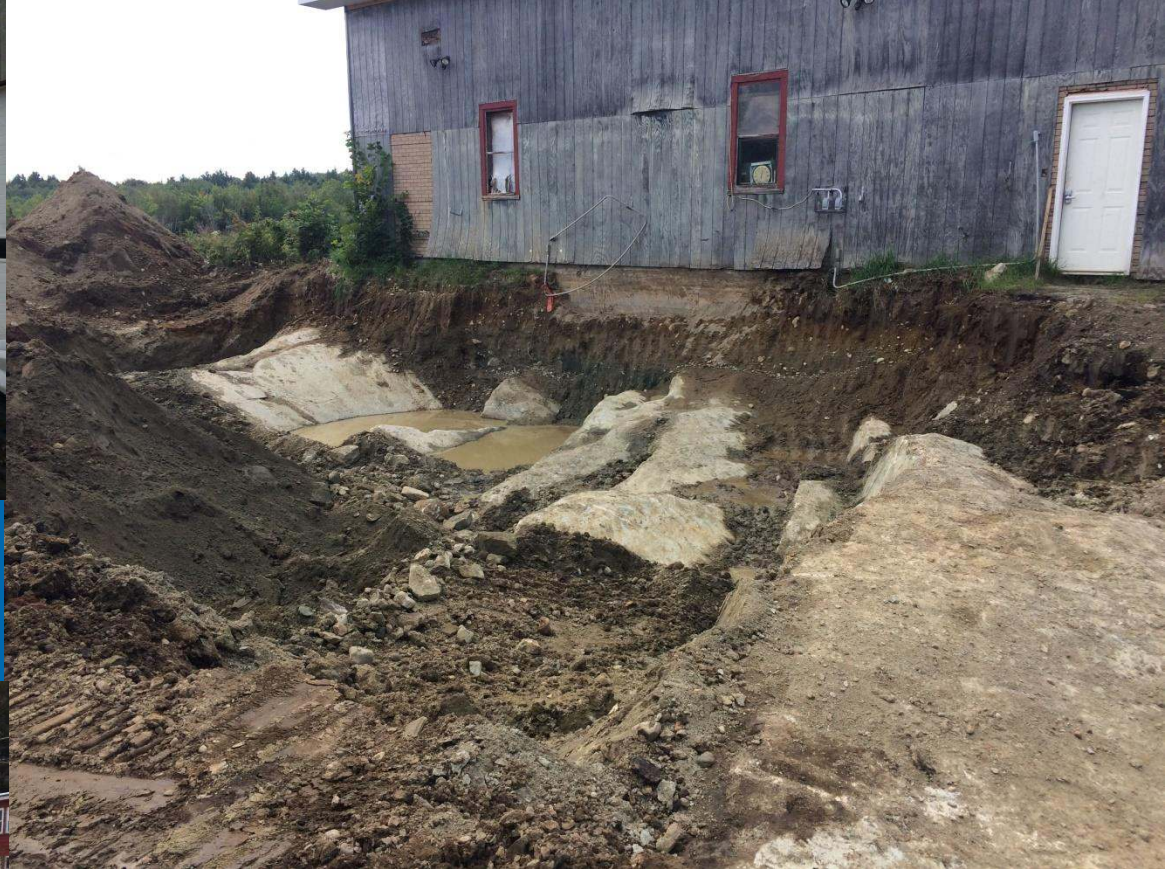
Contaminated soil removal showing bedrock impact on LNAPL migration
