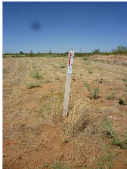
Gas Line Marker on an Infill Lot
