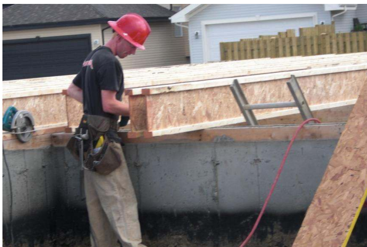
Figure 5: Joist being cut to correct length
