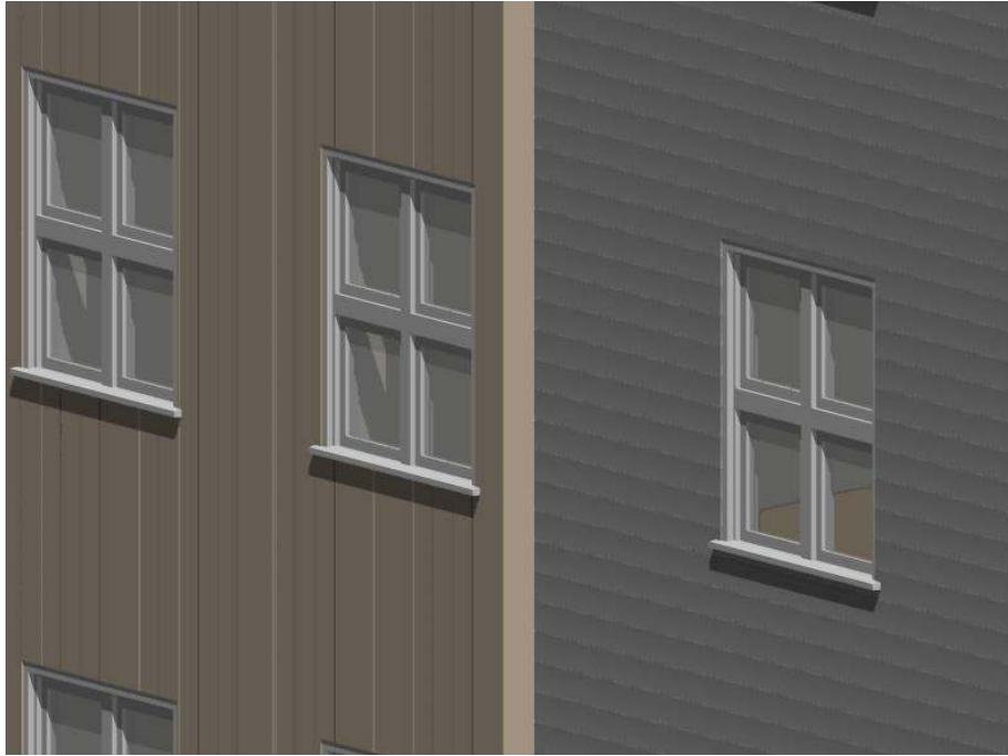
Figure 1: Exterior vertical siding and horizontal siding finishing
