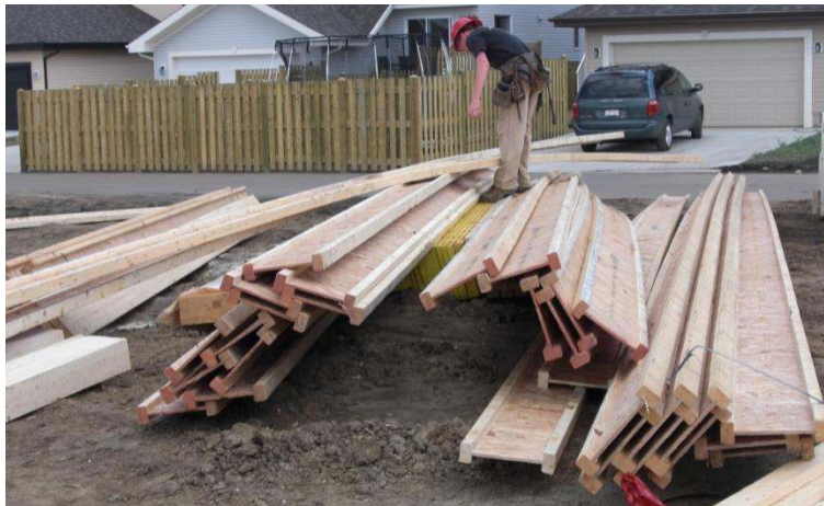
Figure 4: Floor joist package
