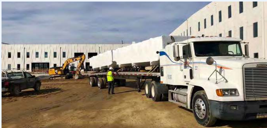
MEP racks were preassembled in a shop about 100 miles away and shipped to the site in 25ft-long 3,000-lb assemblies.
