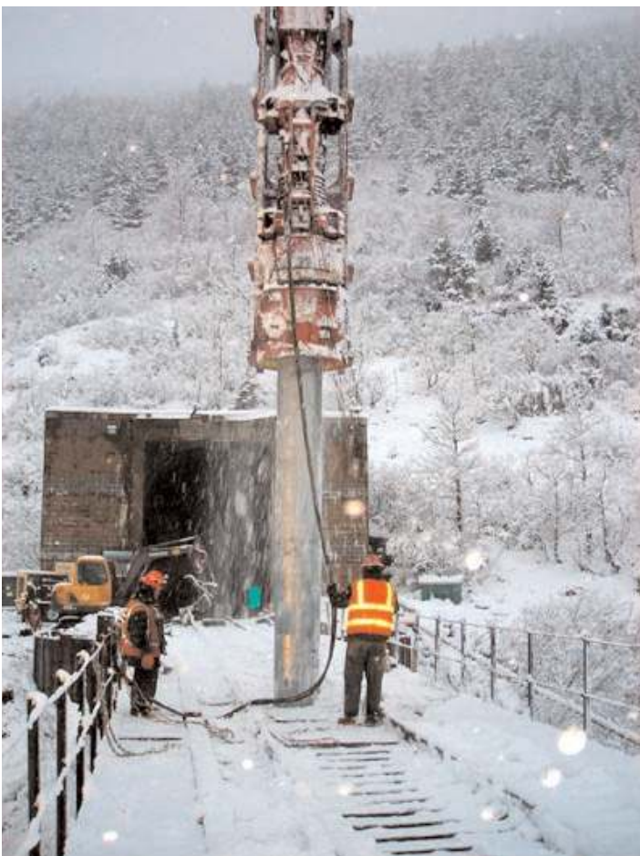
Alaska Railroad Bear Valley Bridge, Portage
