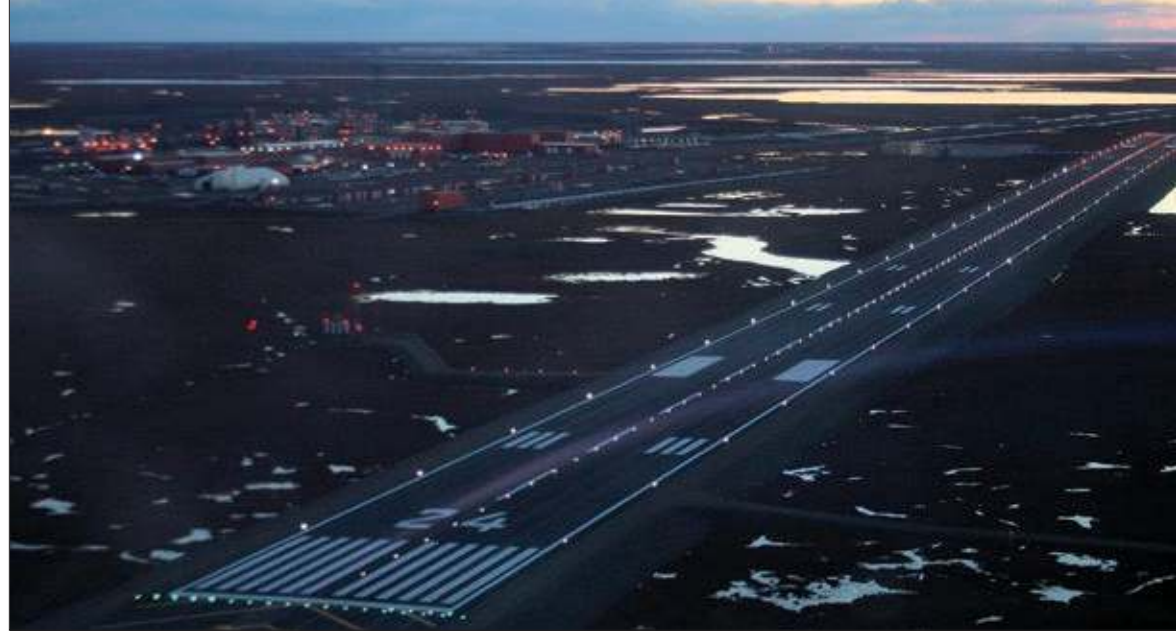
Kuparuk Airfield, Granite Construction
