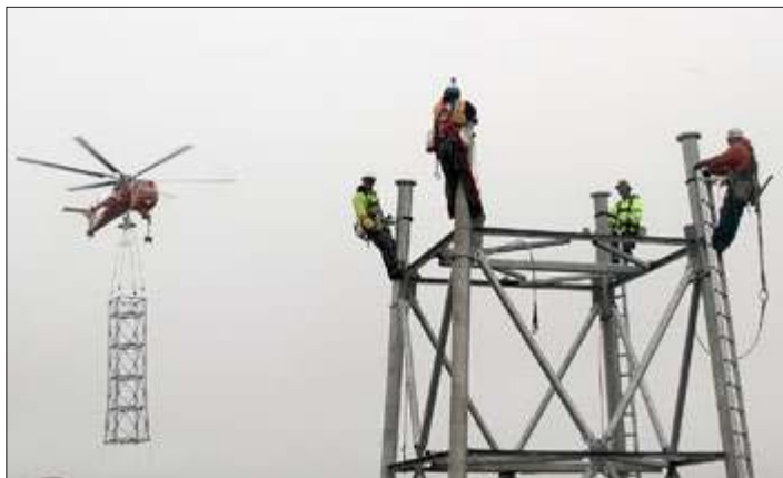
Heavy Lift Tower Section, Yukon River, STG Inc.
