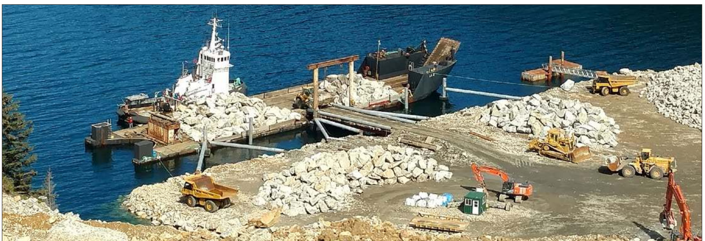
St. George Breakwater Storm Repair, Brice Inc.
