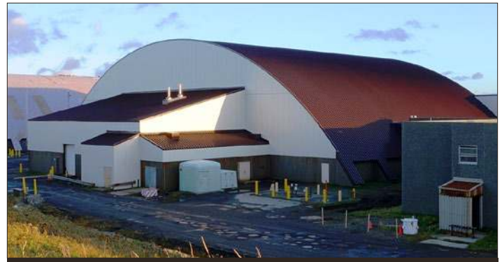
Shemya Eareckson Air Station Roof Repair, Rain Proof Roofing
