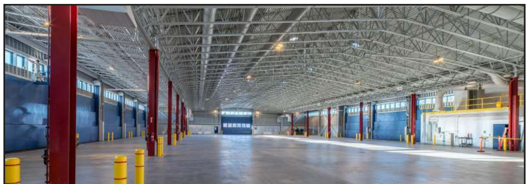
Juneau Snow Removal Equipment Building – F&W Construction Company, Inc.
