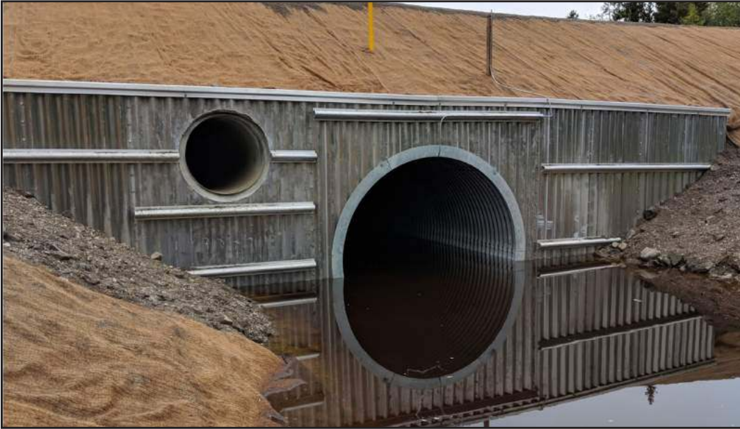
Campion Road Beaver Creek Culvert Replacement – Cruz Construction, Inc.
