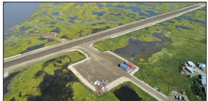
2013 Scammon Bay Airport Flood Permanent Repairs – Brice, Inc.
