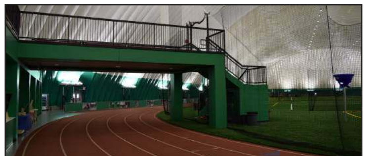
The Dome/Reconstruction – Davis Constructors & Engineers, Inc.
