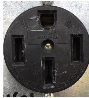
220/50 Amp Outlet. Requires this connection.
