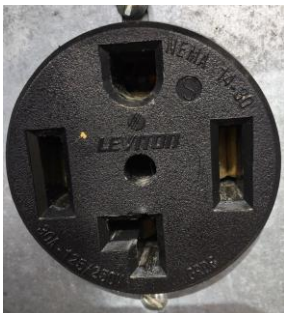
220/30 Amp Outlet. Requires this connection.
