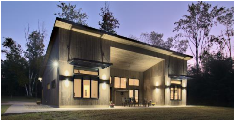
CMB Construction Home #1 – Group A Judge’s Awards: Master Suite, Interior Design, Kitchen, Craftsmanship & Judge’s Overall People’s Choice Award
