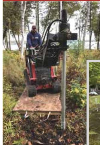
Helical Piers can be installed through wetlands for boardwalk and deck foundations. Beams are attached to brackets for traditional deck framing.
