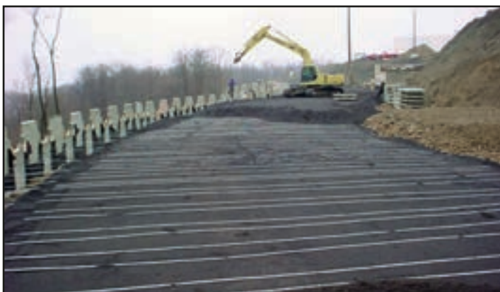
JWC installed a 29,000 square foot reinforced earth retaining wall in addition to performing all site excavation, grading, storm drainage, water, and sanitary sewer installation at the Fort Steuben Mall in Steubenville, Ohio.
