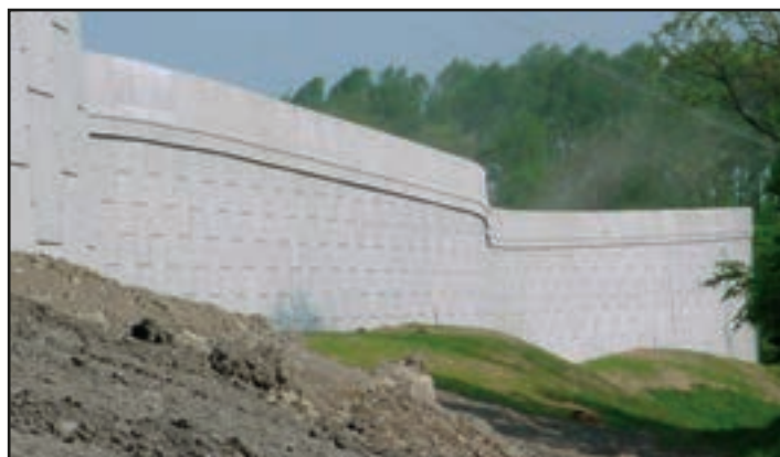
JWC installed a 29,000 square foot reinforced earth retaining wall in addition to performing all site excavation, grading, storm drainage, water, and sanitary sewer installation at the Fort Steuben Mall in Steubenville, Ohio.
