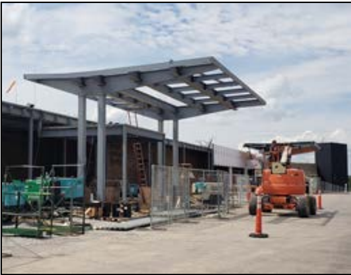
New main and emergency room entrances were constructed and included overhangs for coverage during patient drop-offs. Contractors also constructed a new front corridor, shown completed in the photo on the right.
