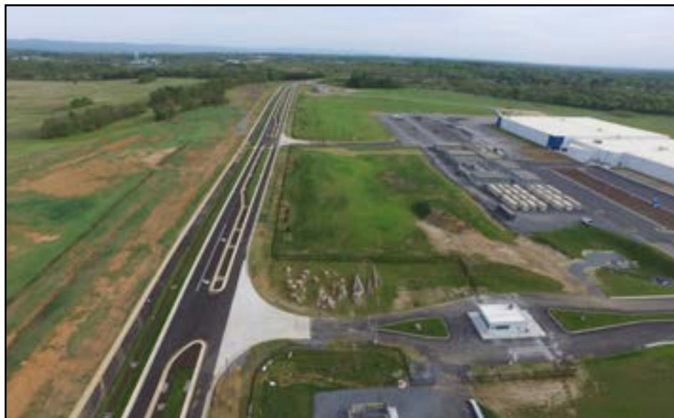
Jefferson Asphalt Products Company, Charles Town, constructed Northport Avenue to serve the plant. Roads and parking lots utilized 68,000 square yards of asphalt.
