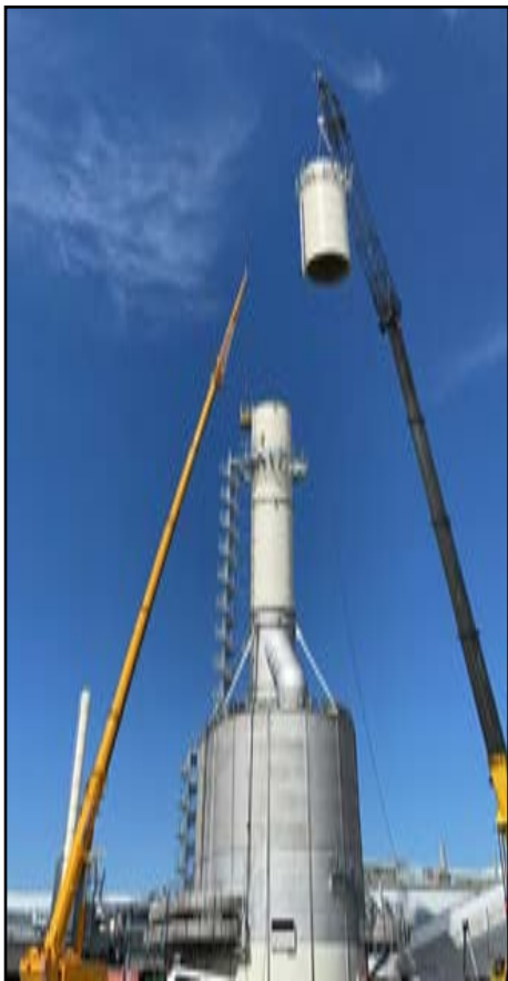
Three chimneys were constructed at the facility; a 213-foot chimney associated with Wet Electrostatic Precipitator or WESP; a 213-foot Aquila furnace chimney; and a 114-foot dedusting chimney – to treat all flue gasses.
