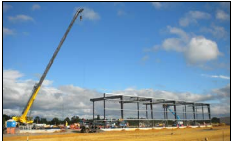
The facility was a design-build project with multiple structures that are a combination of steel and masonry framed structures. There are 2,500 tons of steel in the plant.
