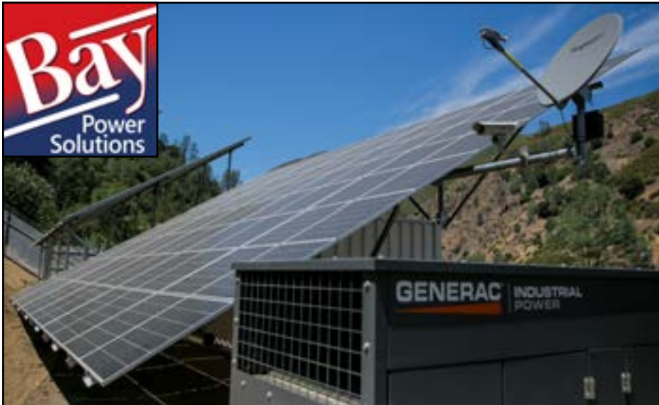
A microgrid based on a gen-set from Generac. (Photo: Bay Power Solutions)
