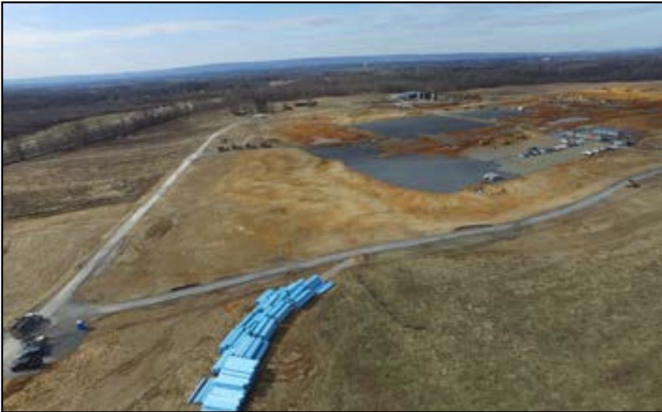
Construction began in late 2017. ALL Construction, Inc., Mt. Storm, performed the initial site preparation and site piping. The new manufacturing facility sits on a 136-acre parcel of land that required 250,000 cubic yards of excavation and 9,000 feet of in-ground stormwater and sewer pipe.
