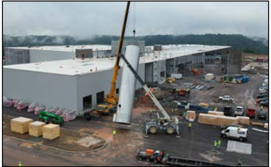
March-Westin Company, Inc. set the 65' reverse osmosis water silo storage tank. The tank weighs approximately 34,500 lbs. (empty) and will hold 50,000 gallons.
