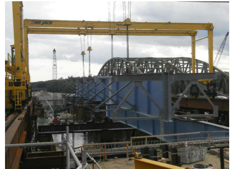
Whittier Memorial Bridge, Newburyport and Amesbury, MA
