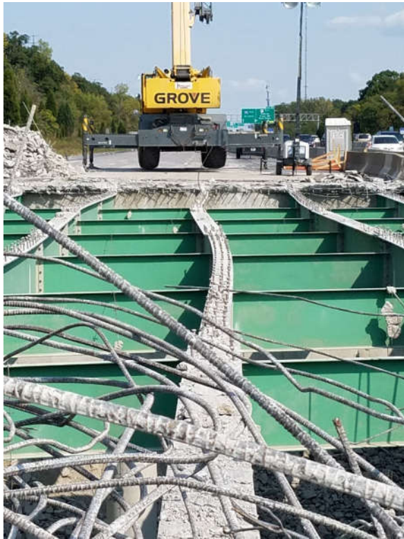
I470 Bridge Re-decking, Kansas City, MO
