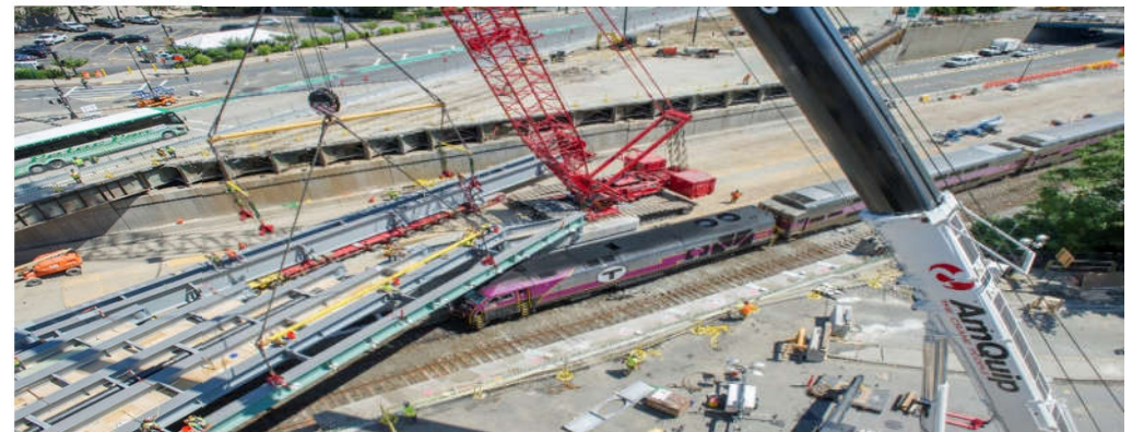
Comm. Ave Bridge, Boston, MA
