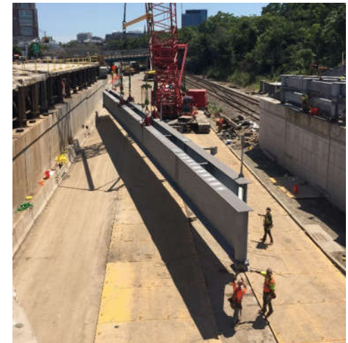
Comm. Ave Bridge, Boston, MA
