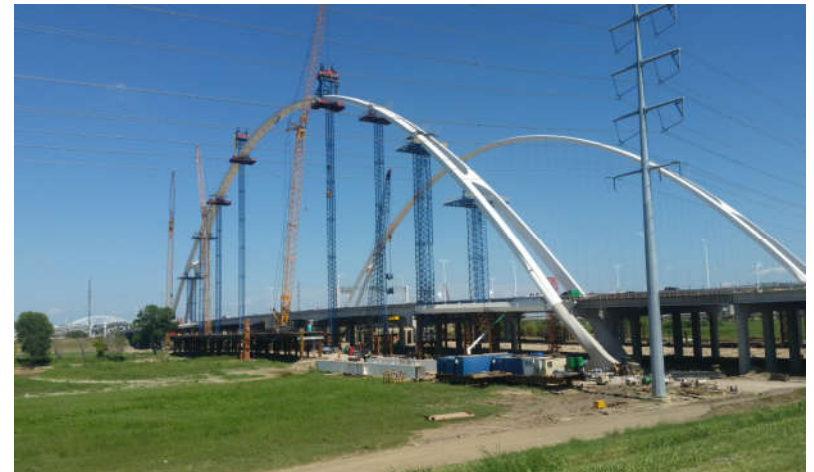
Margaret McDermott Bridge, Dallas, Tx.
