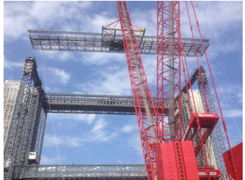
Fore River Lift Span Demolition, Quincy, MA
