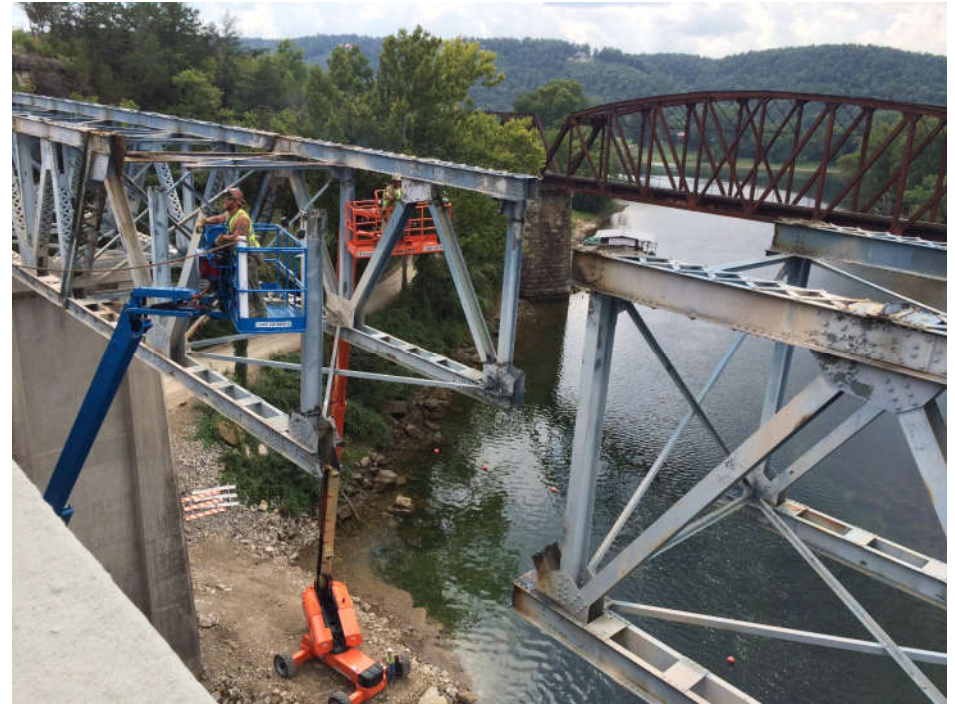
White River Truss Demolition, Prairie County, AR
