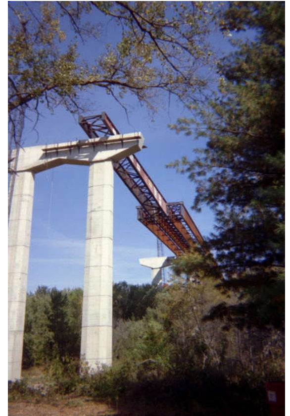
US 20 – Iowa River Bridge
