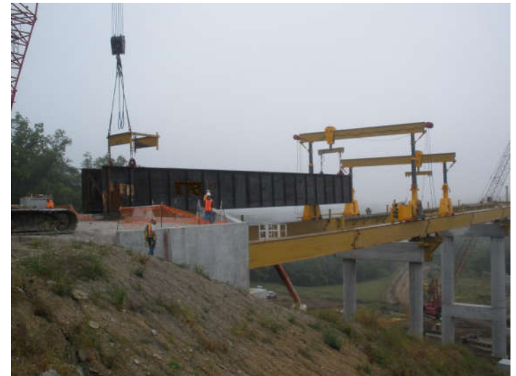
Kate Shelly Replacement Bridge, Boone, IA
