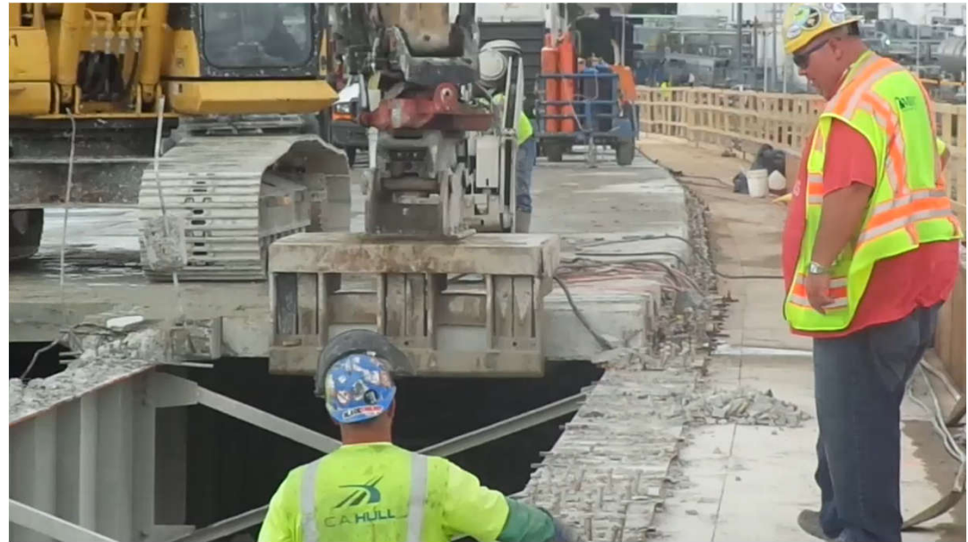
I-75 Deck Replacement, Detroit, MI
