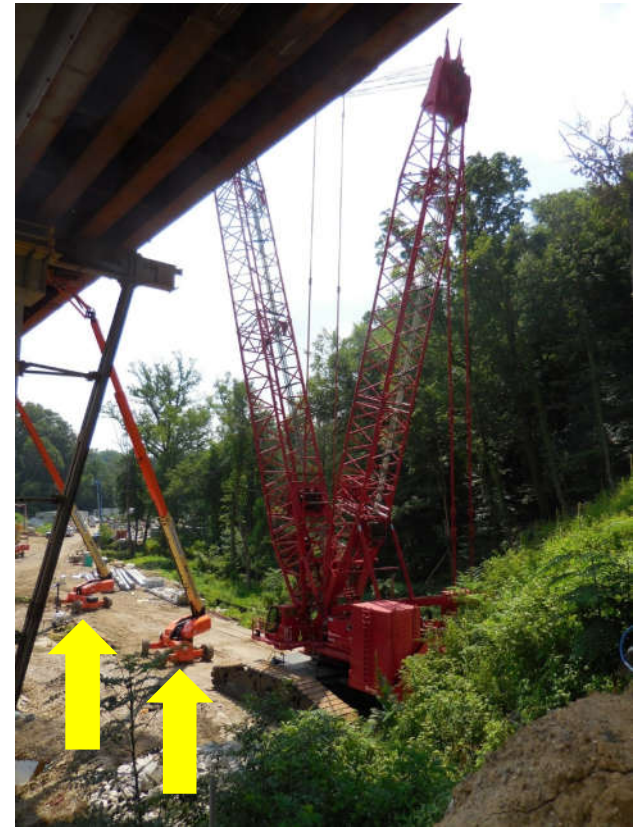
Crum Creek Viaduct, Swarthmore, PA
