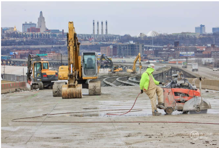
Lewis and Clark Viaduct, Kansas City, MO
