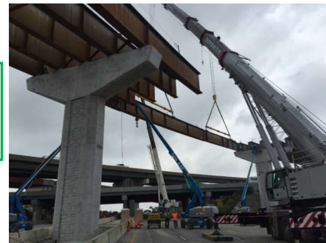
Gateway Interchange Flyovers, Johnson County, KS
