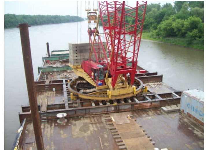
South Omaha Bridge – 4100 Ringer Crane
