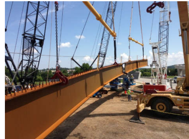
Fulbright Expressway, Fayetteville, AR
