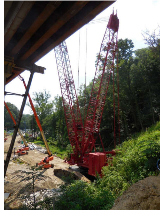
Crum Creek Viaduct, Swarthmore, PA
