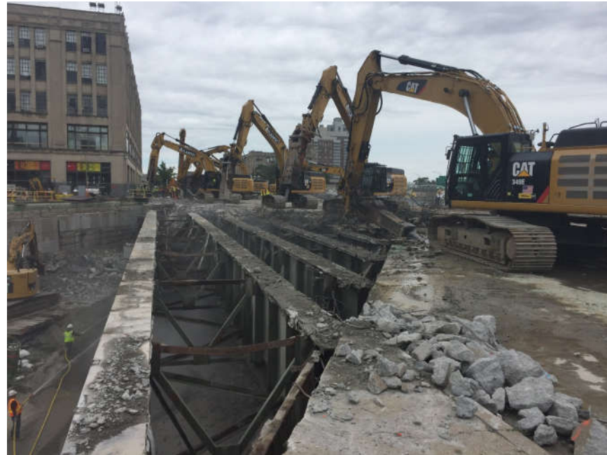
Comm. Ave Bridge, Boston, MA
