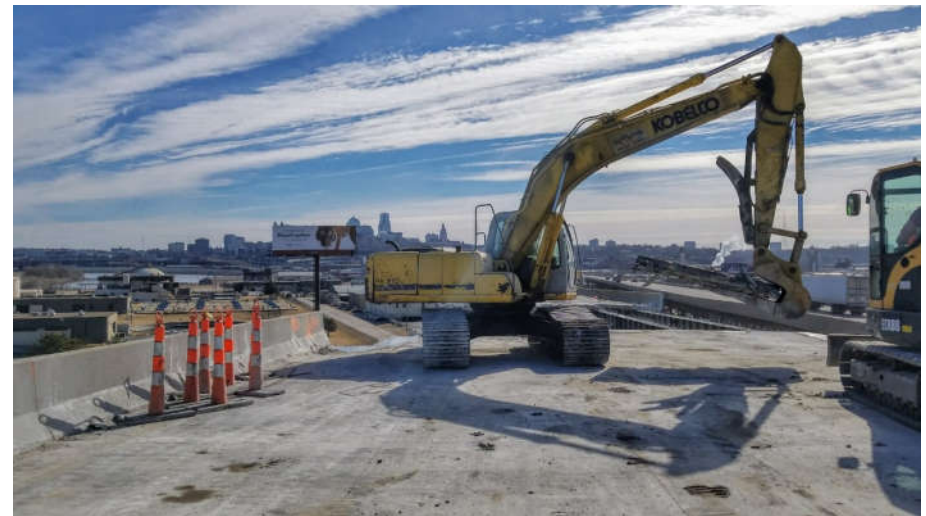
Lewis and Clark Viaduct, Kansas City, MO
