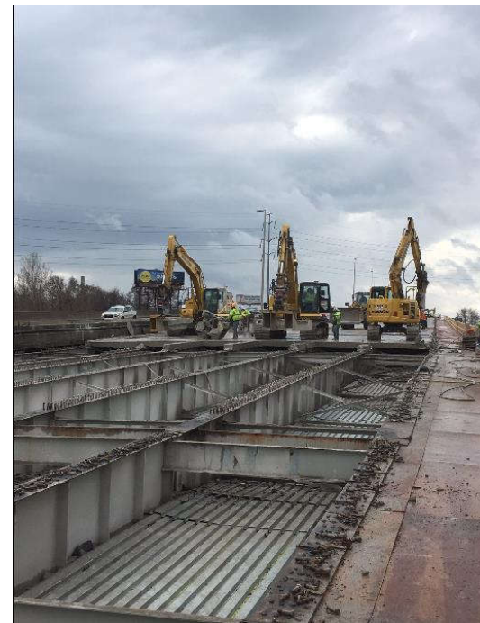
I-75 Deck Replacement, Detroit, MI
