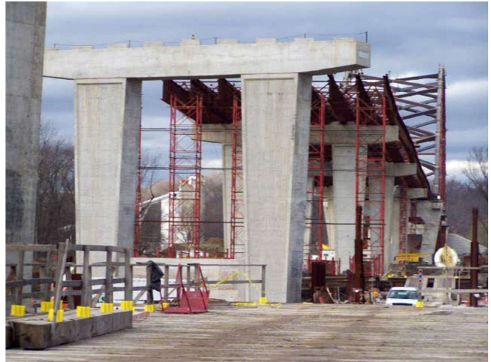
Blennerhasset Island Bridge, Parkersburg, WV
