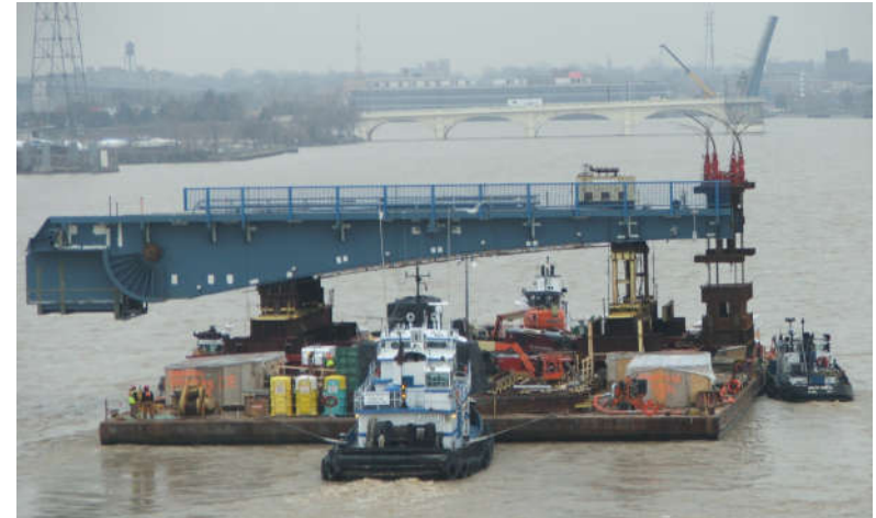
MLK Bridge Replacement, Toledo, OH
