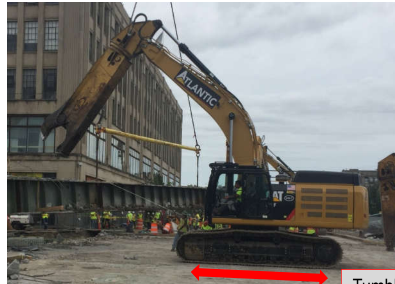
EXCAVATOR CAT 349 (120,000 lb) On a partially composite to noncomposite structure
