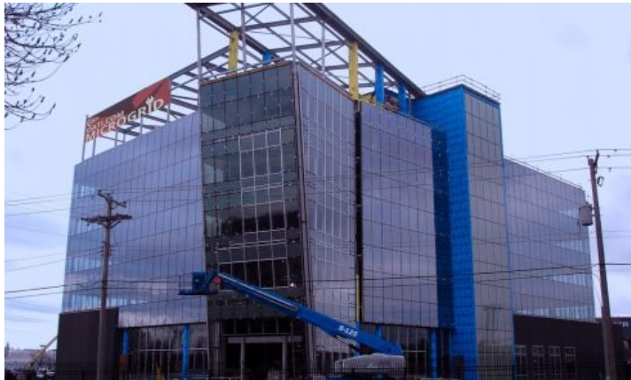
OATI OFFICE BUILDING - BLOOMINGTON, MN
