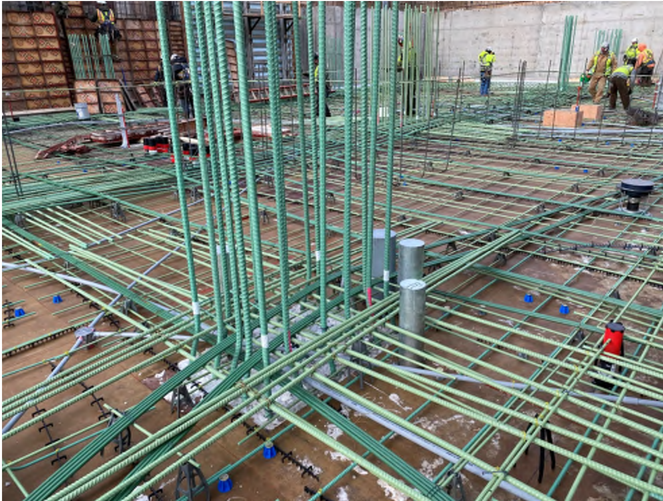
EPOXY COATED REINFORCING STEEL AT EXPOSED AREAS
