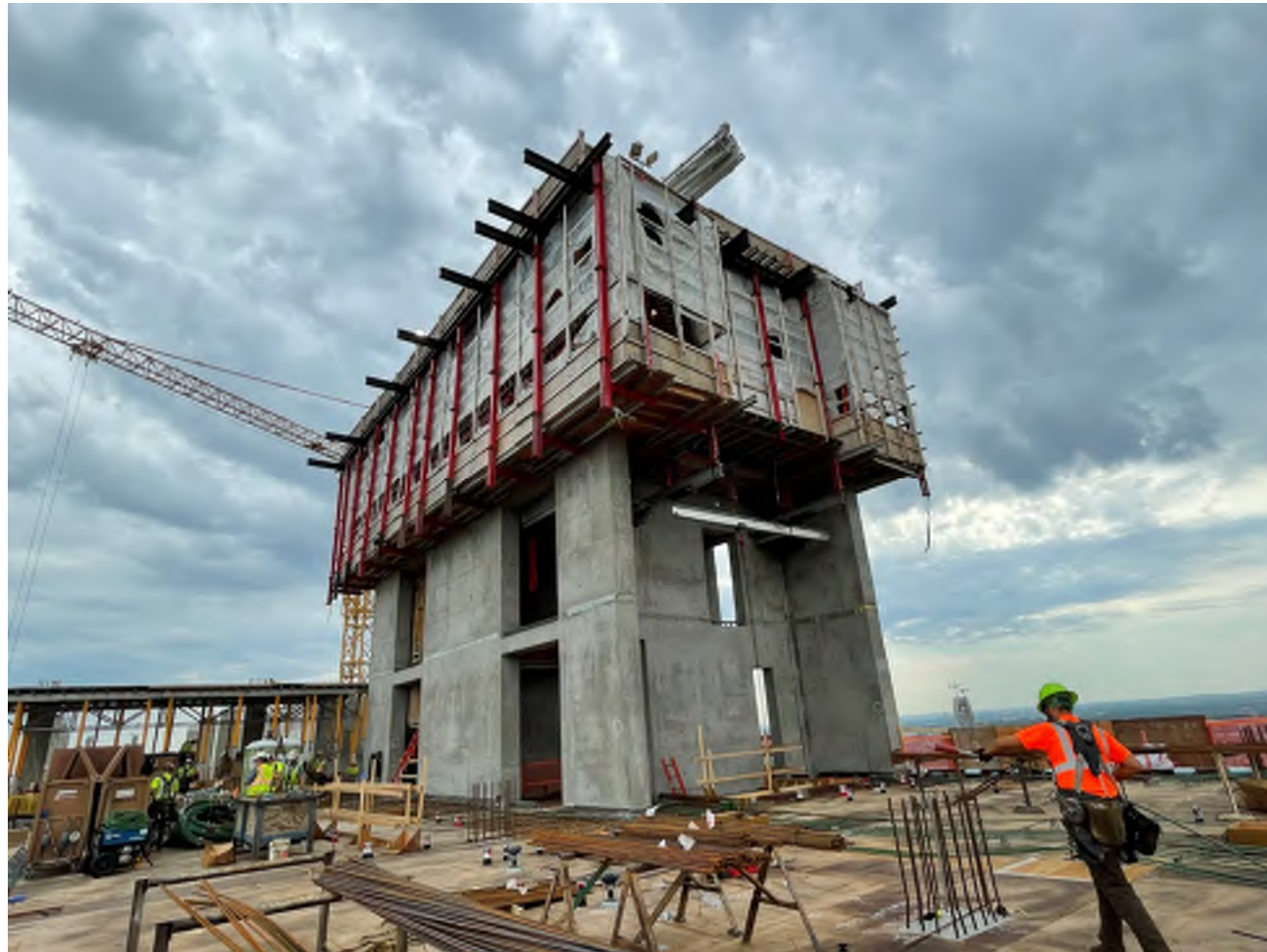
SLIP FORMING FOR CONCRETE SHEAR WALL CORES
