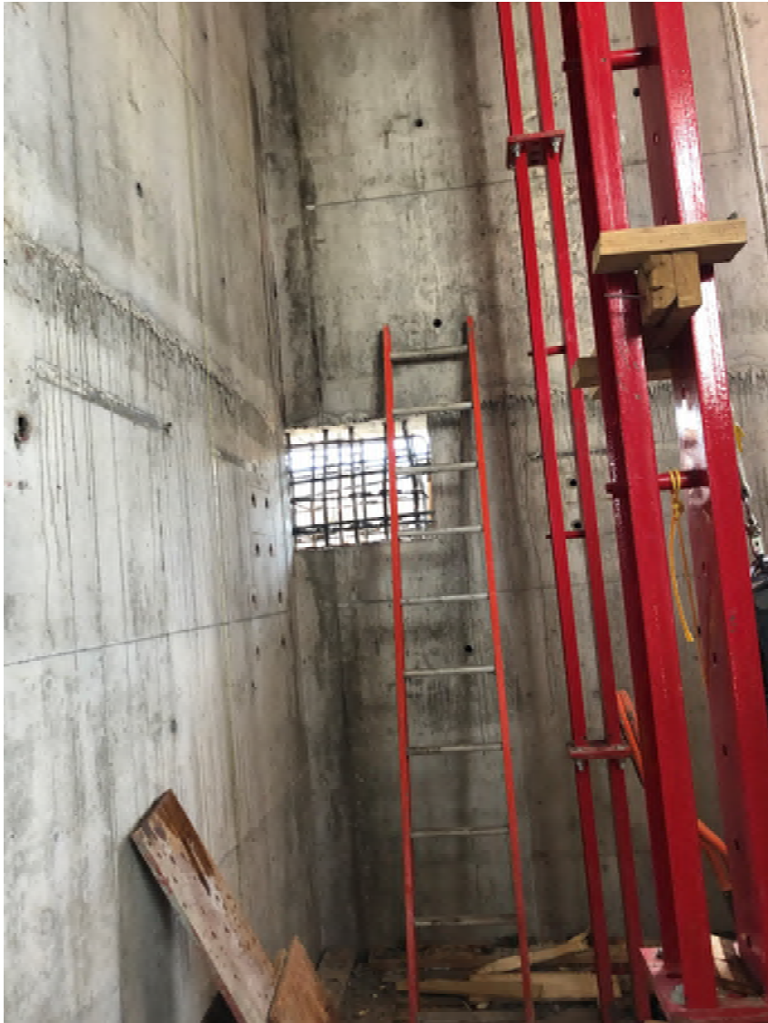
Beam pocket and core system
