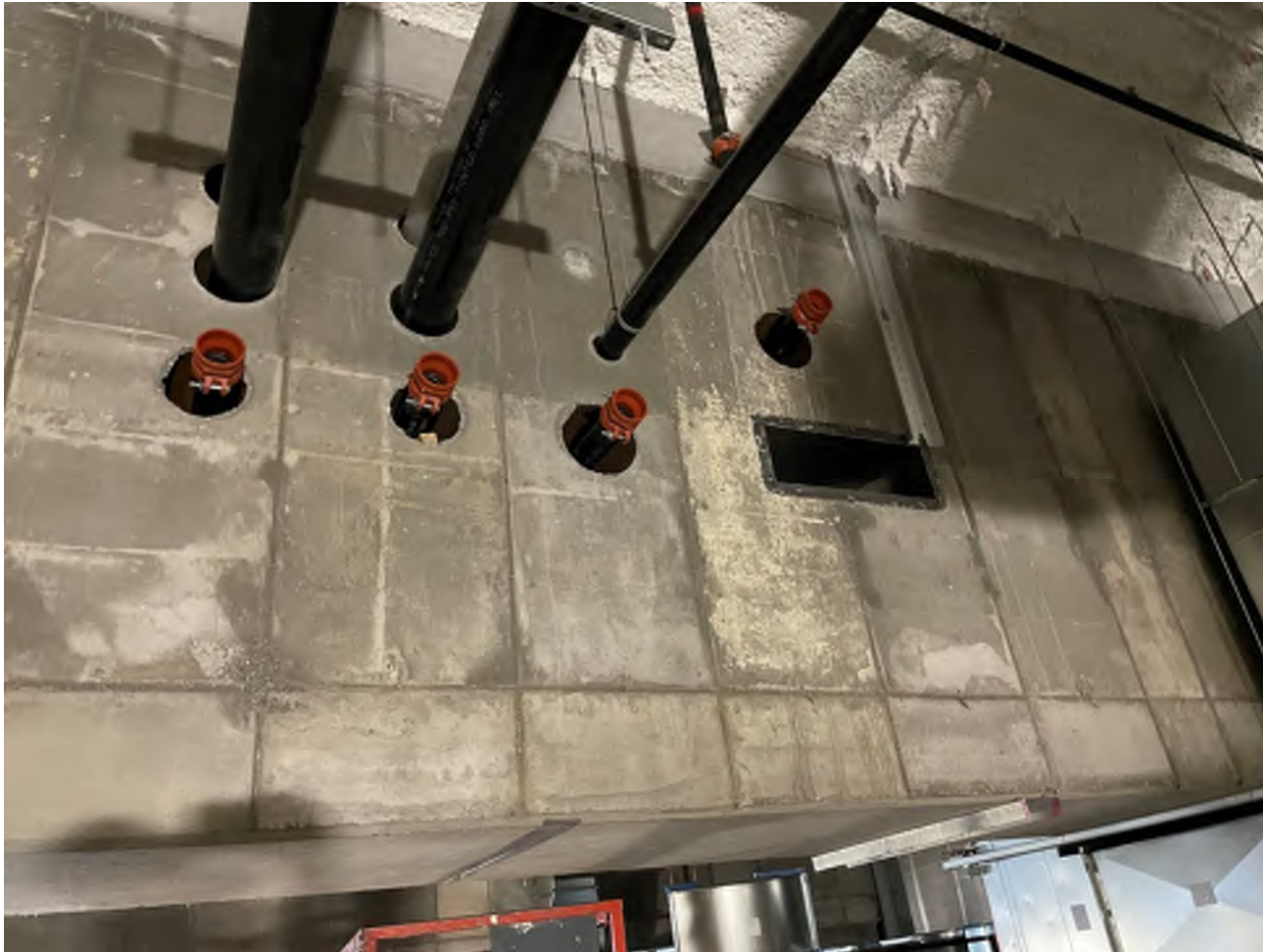
PENETRATIONS IN A TRANSFER BEAM
