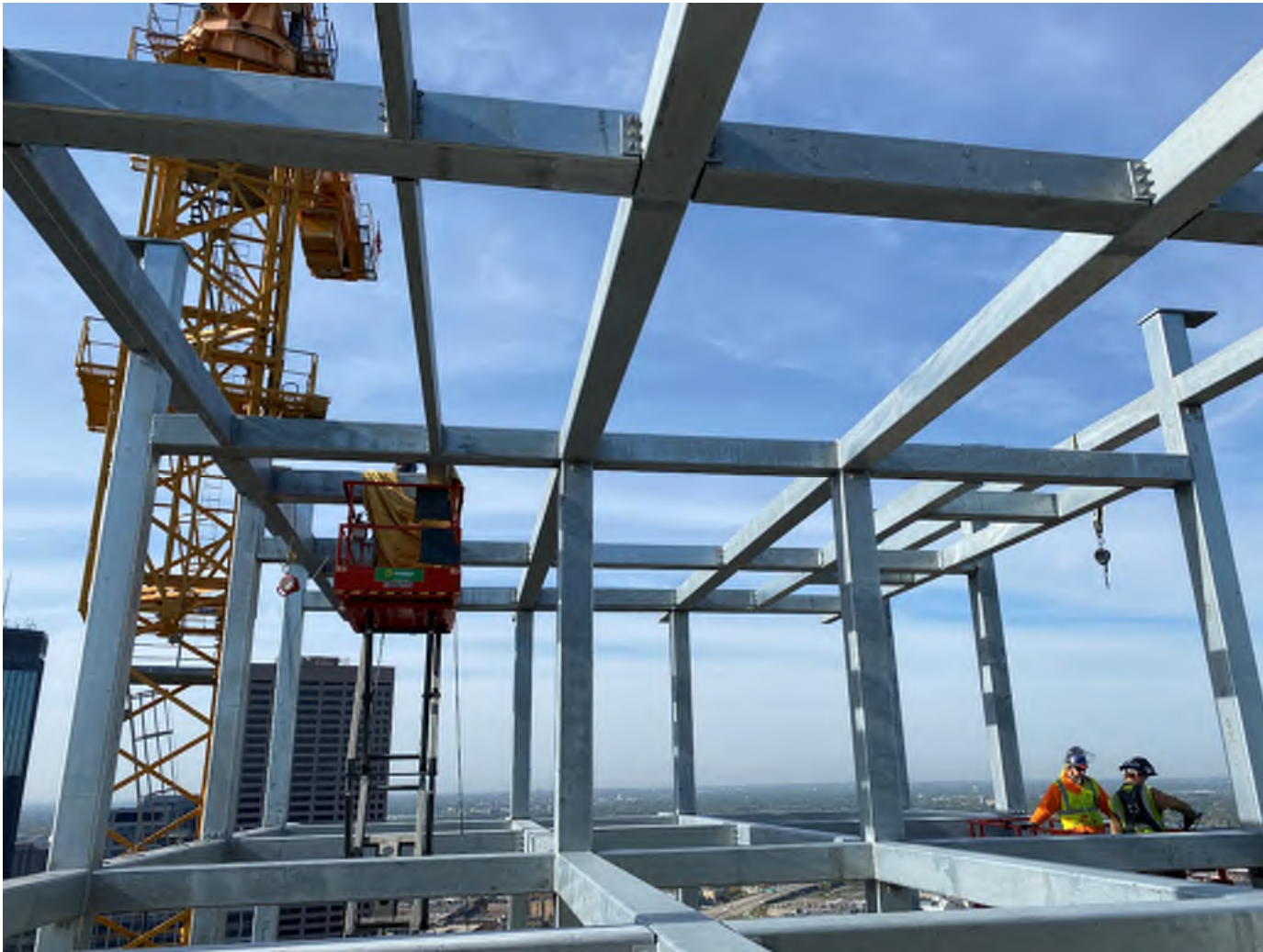
HSS FRAMING AT THE TOP OF THE BUILDING
