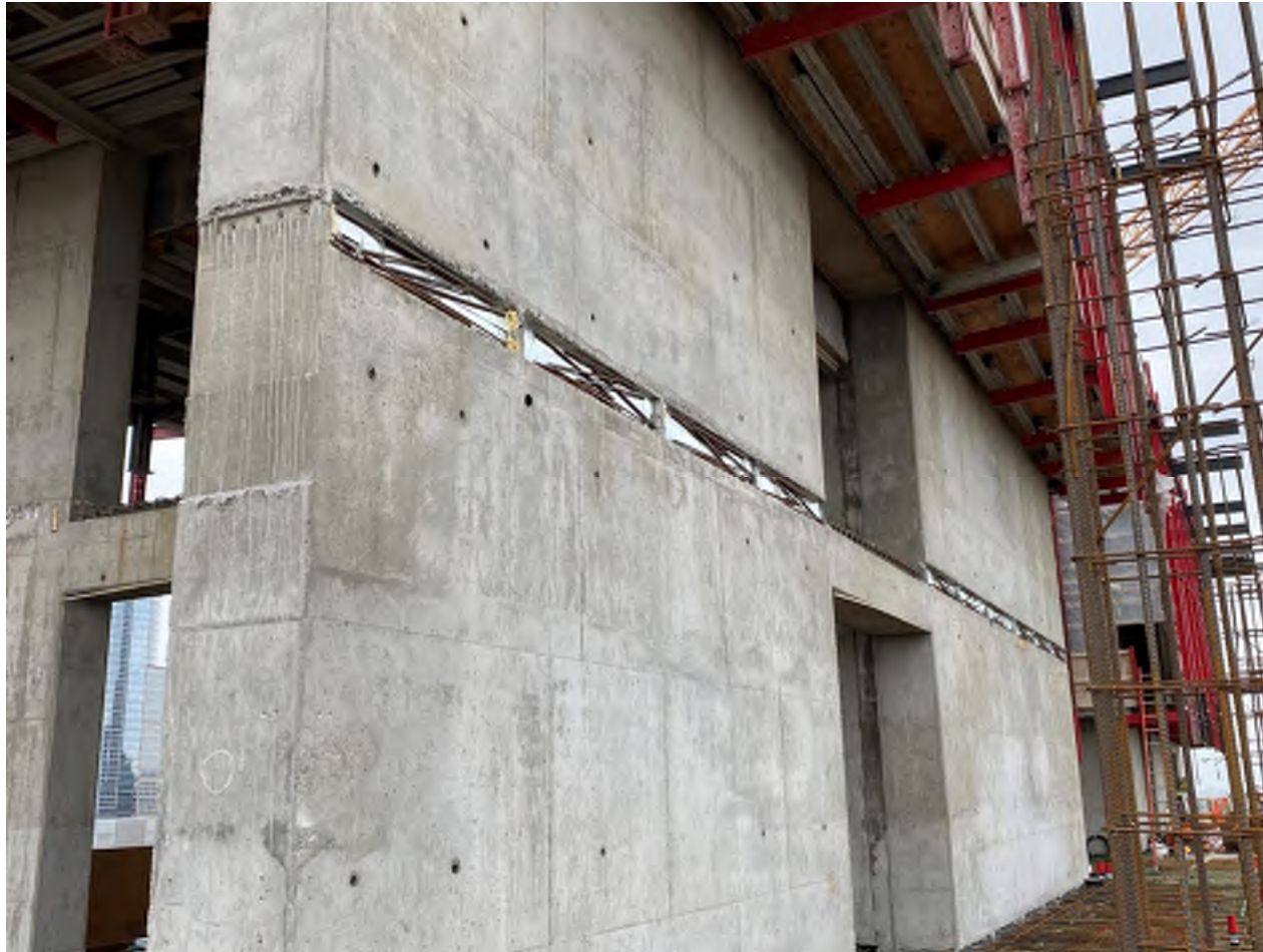
STAYBOX REBAR SYSTEM FOR SLAB DOWELS
