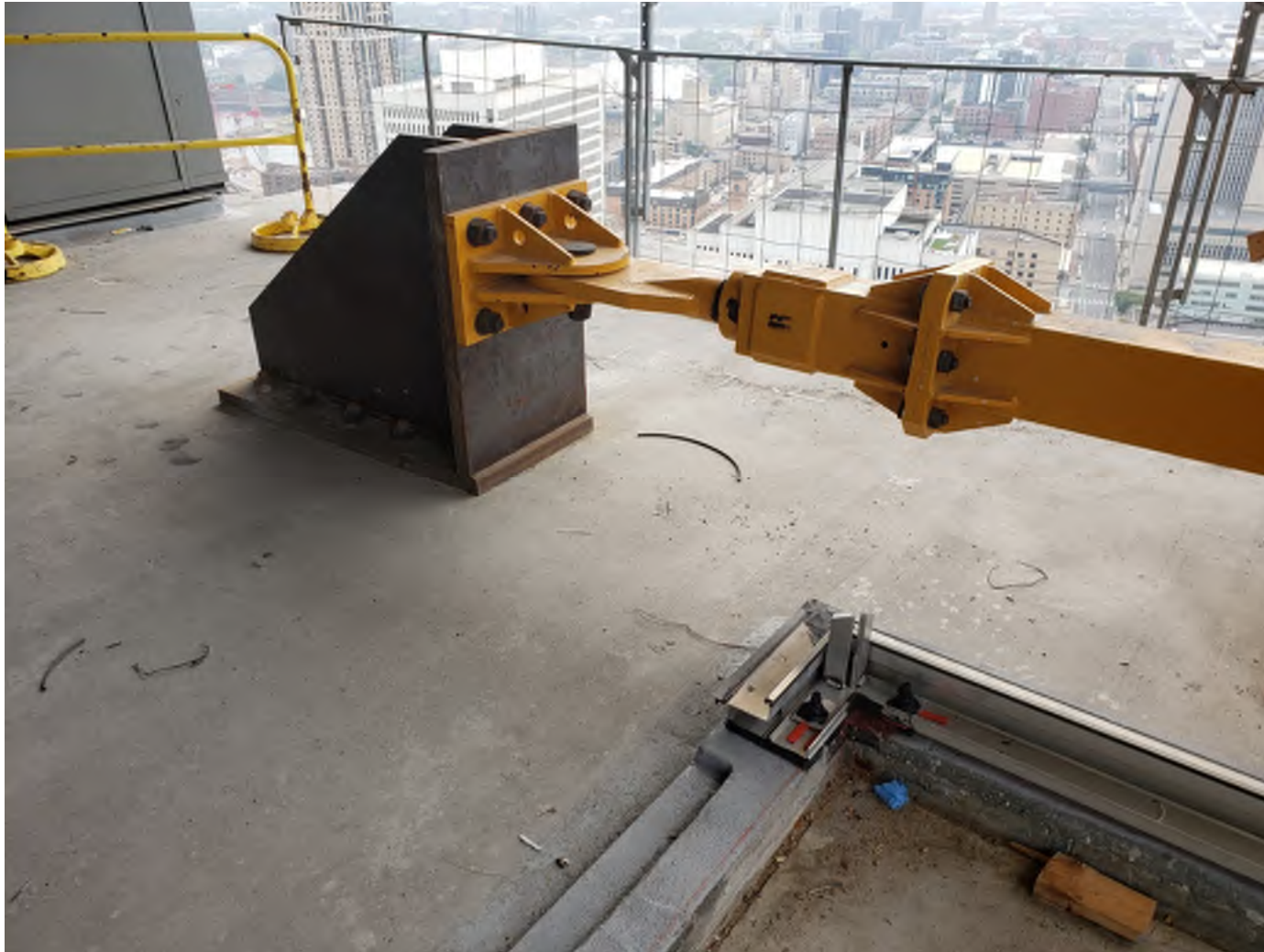
TOWER CRANE TIE-IN
