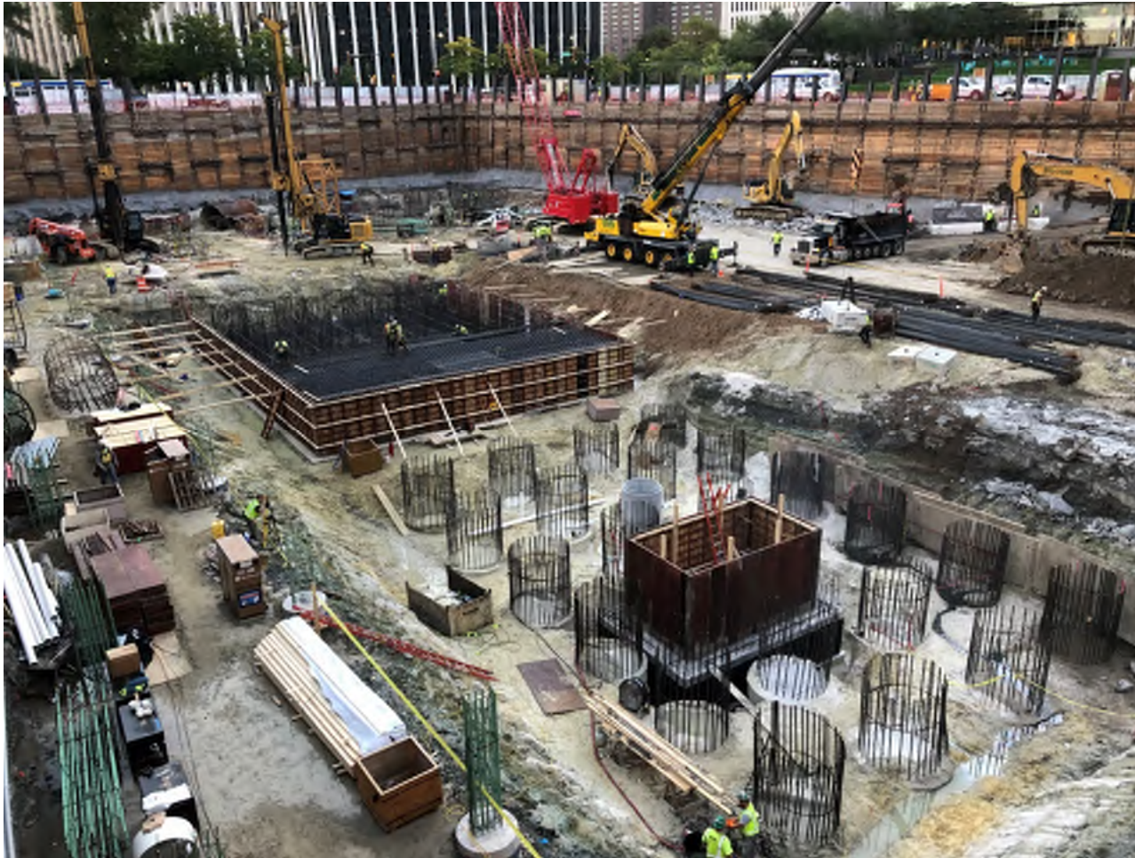
MAT AT SHEAR WALL CORE 8 FEET THICK
