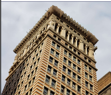
Steel framing, terra cotta cornice
