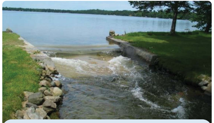
The new outlet structure, with its V-shaped weir, newly opened, June 25, 2005.
