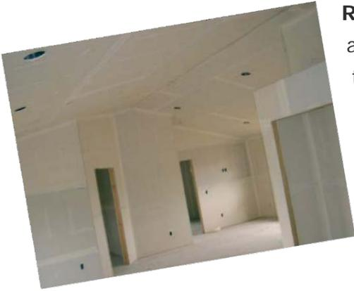
**Residential contractors** install heat and sound insulation, ceilings, and interior walls in single-family homes. Walls and ceilings are typically made from various types of gypsum panels nailed into place over wood framing installed by the builder. Various finishing work hides joints and prepares the surfaces for painting. Insulation materials typically are fiberglass pads and foam panels but may also be sprayed or loose materials like cellulose.
