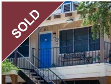
Courtney Place, 221 units
