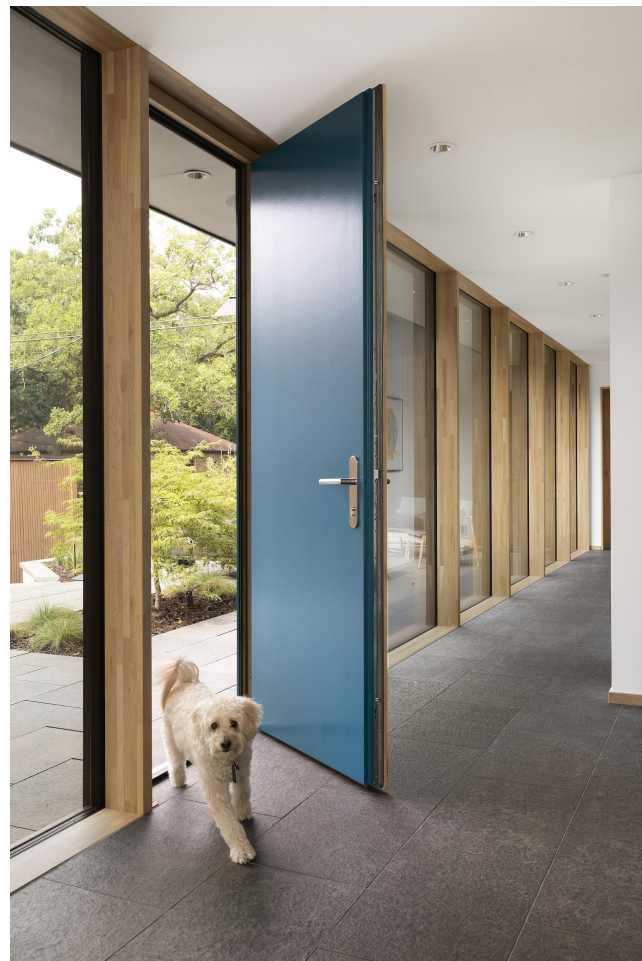
TOP & RIGHT: Images show undeniable connection between the inside and outside spaces. The stone tiles selected by the client are flamed and brushed basalt and are the same inside and outside the home. The inside tiles are installed with a 3/16" grout joint whereas when outside they were installed with a 3/16" wide open joint to allow permeability.
