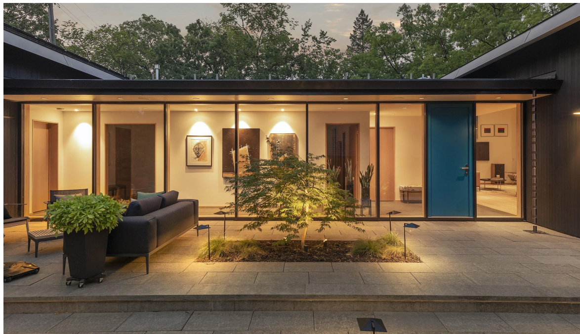
TOP & RIGHT: Images show undeniable connection between the inside and outside spaces. The stone tiles selected by the client are flamed and brushed basalt and are the same inside and outside the home. The inside tiles are installed with a 3/16" grout joint whereas when outside they were installed with a 3/16" wide open joint to allow permeability.
