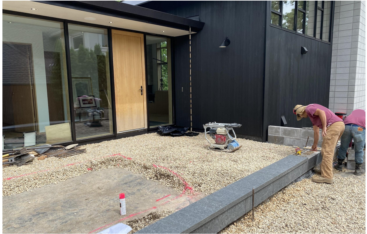
LEFT: Images are “before” images showing the entry patio area. Permitting required that the patio and sidewalk be constructed as permeable hardscapes..
