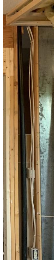
DURING-RELOCATED WASTE STACK
