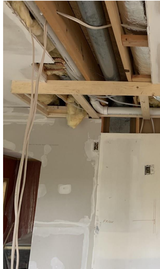
DURING-RELOCATED VENT AND WATER LINES
